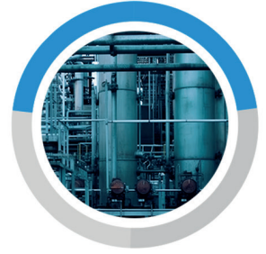
Kap Kazan Sanayi Cap Boiler Industry
